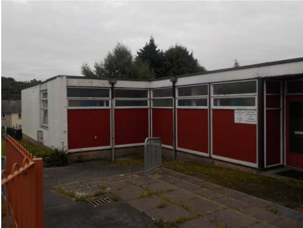
Flat roof sections of the school buildings
